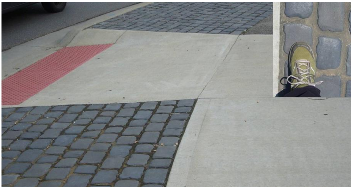
Figure 4-10: Example of surface material that was not recognized as a non-walking surface by blind participants
