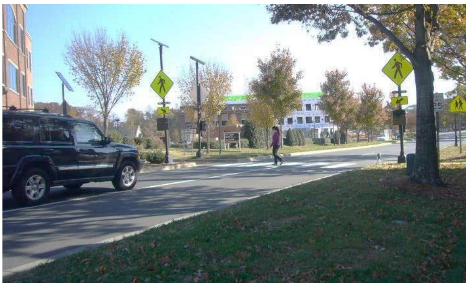
Figure 5-13: RRFB at Two-Lane Roundabout
