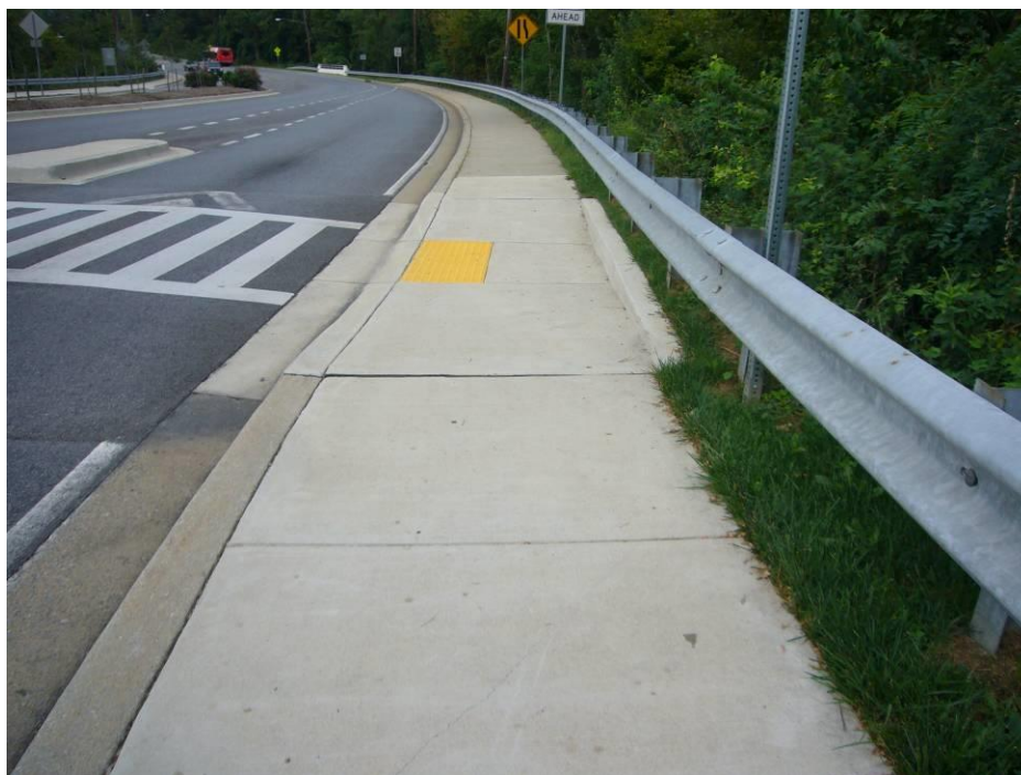
Figure 4-16: Image of Parallel Curb Ramp
