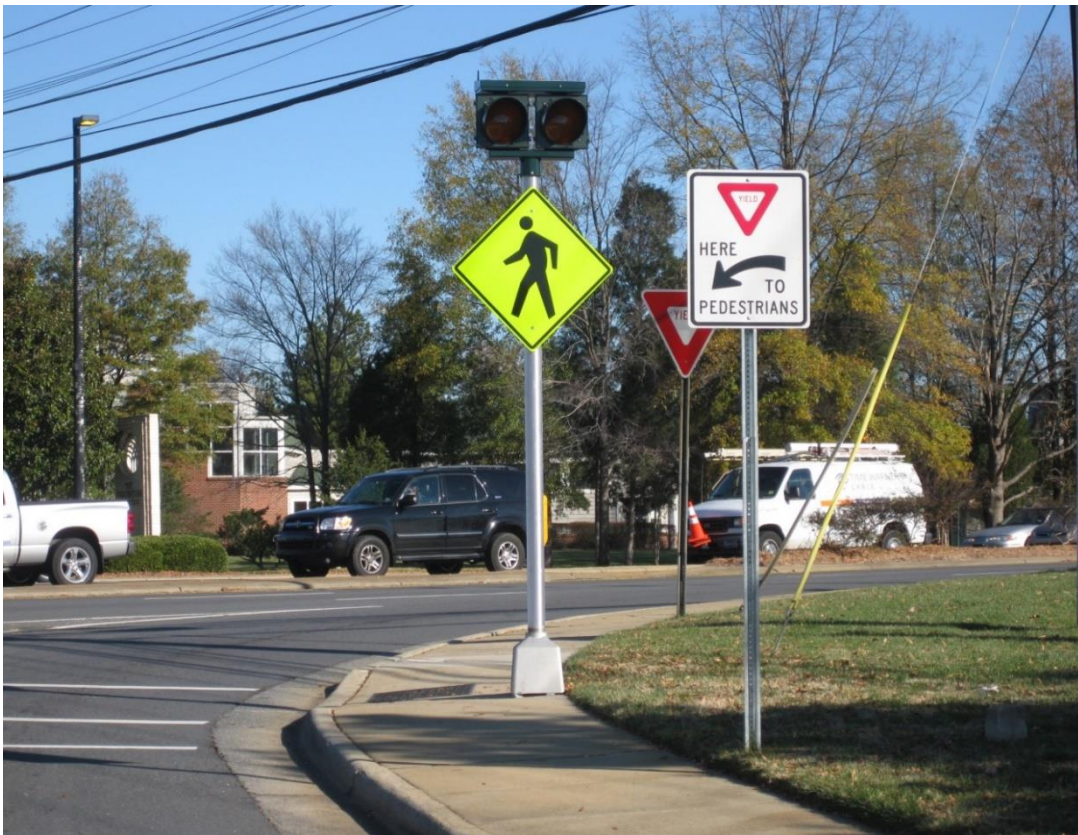
Figure 10-6: Flashing beacon at CTL
