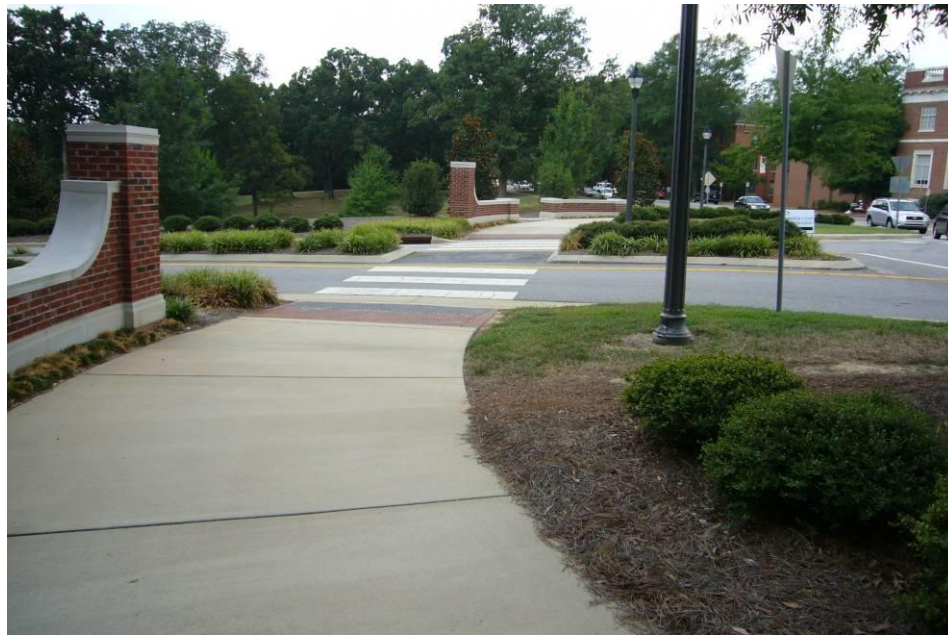
Figure 4-8: Sidewalk curving away from the corner to guide pedestrians directly to the crosswalks
