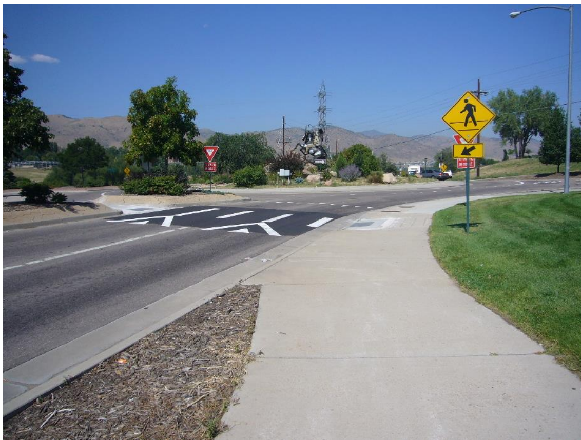
Figure 10-4: Raised Crosswalk at two-lane roundabout
