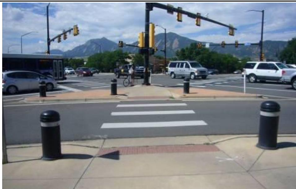
Figure 5-14: Detectable warning surfaces installed at a CTL crossing
