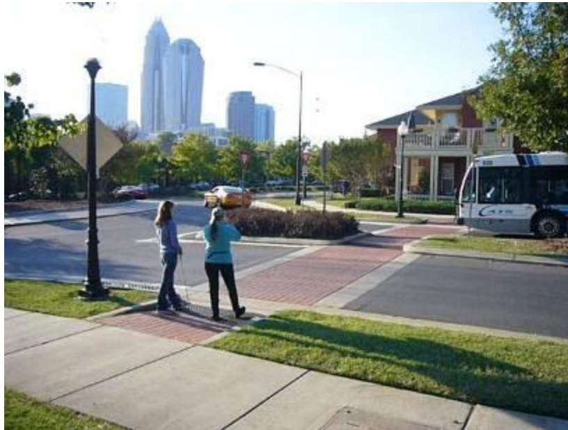
Figure 4-15: Curb ramp with returned curbs
