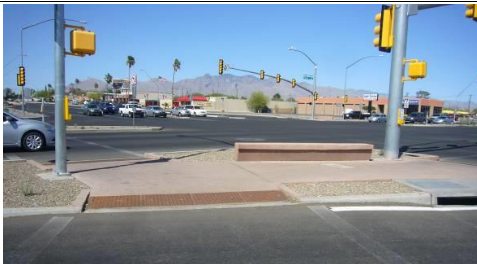
Figure 5-5: Island with ramps to paved walkways and gravel outside pedestrian path area
