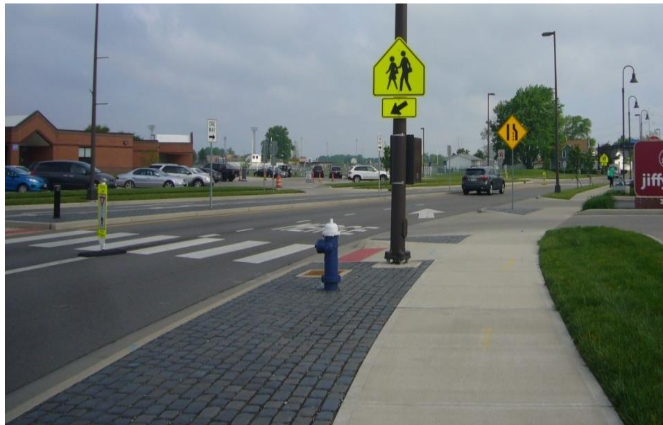
Figure 3-7: Sidewalk separation at roundabouts not detectable
