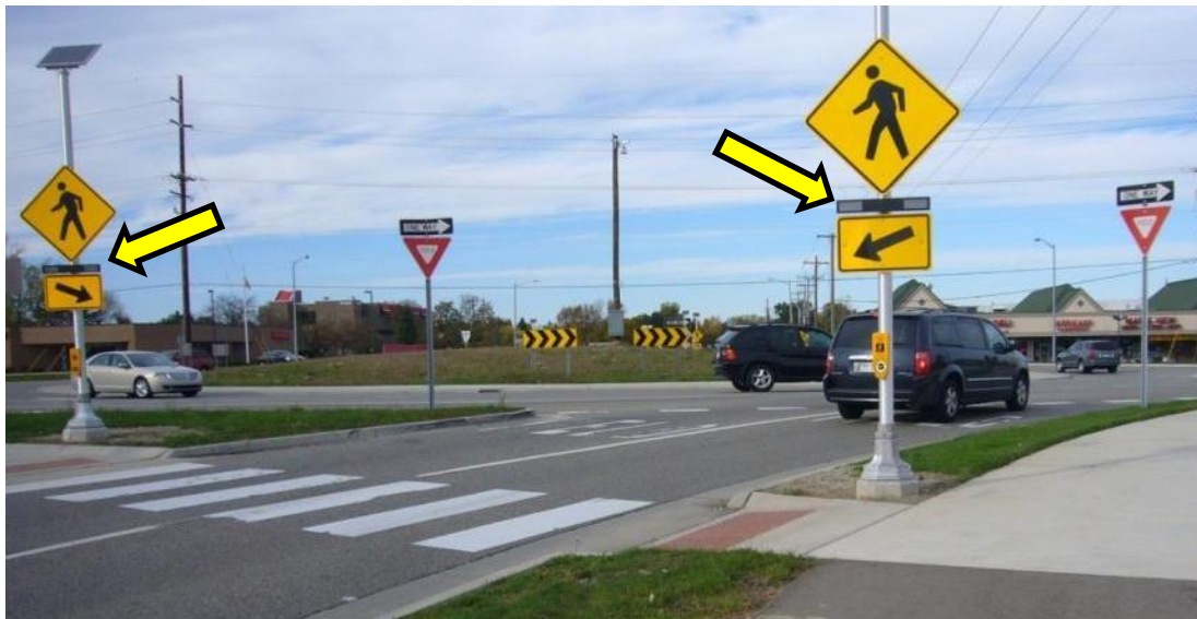
Figure 4-24: Rectangular Rapid Flash Beacon at roundabout in Oakland County, Michigan
