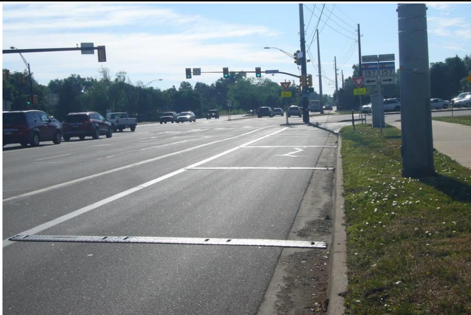
Figure 5-17: Sound Strips installed at Channelized Turn Lane
