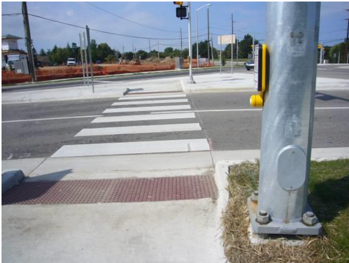
Figure 5-16: Pushbuttons with pushbutton locator tones assist with locating the crosswalk and maintaining correct heading while crossing
