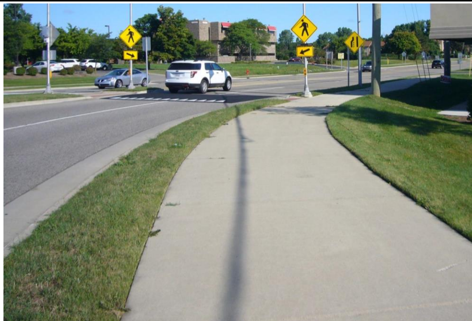
Figure 3-5: Detectable landscape separation at roundabouts
