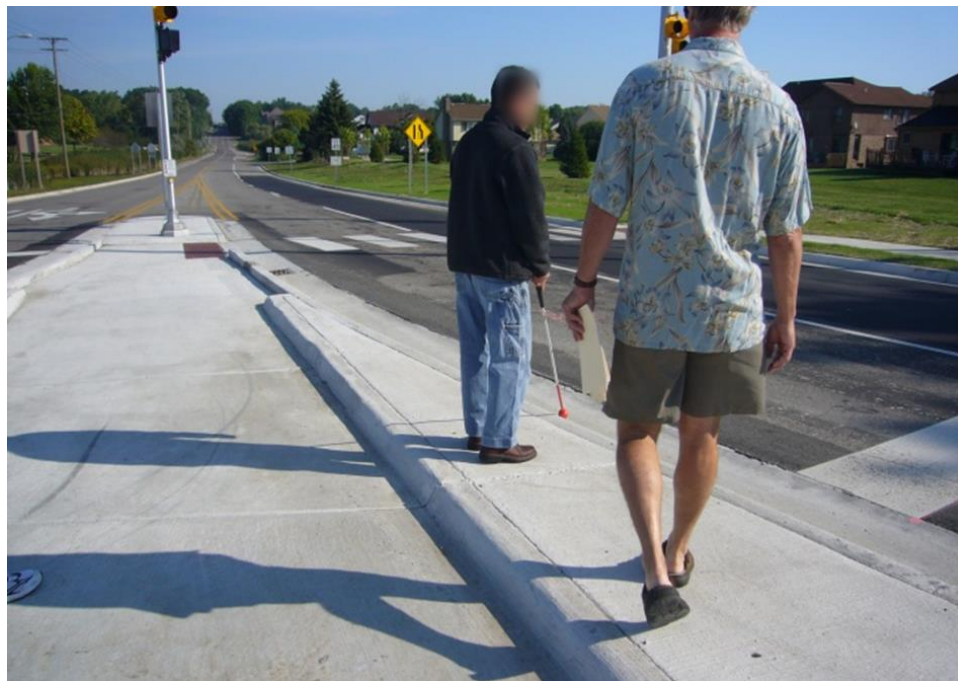
Figure 4-18 Image of all paved roundabout splitter island
