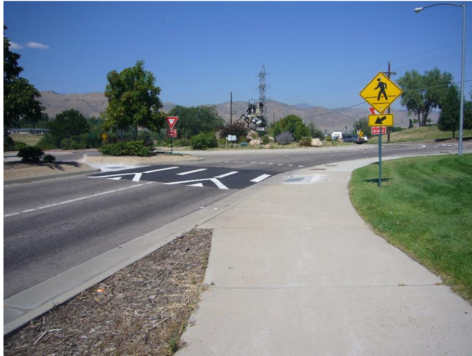
Figure 4-29: Raised Crosswalk at Two-Lane Roundabout
