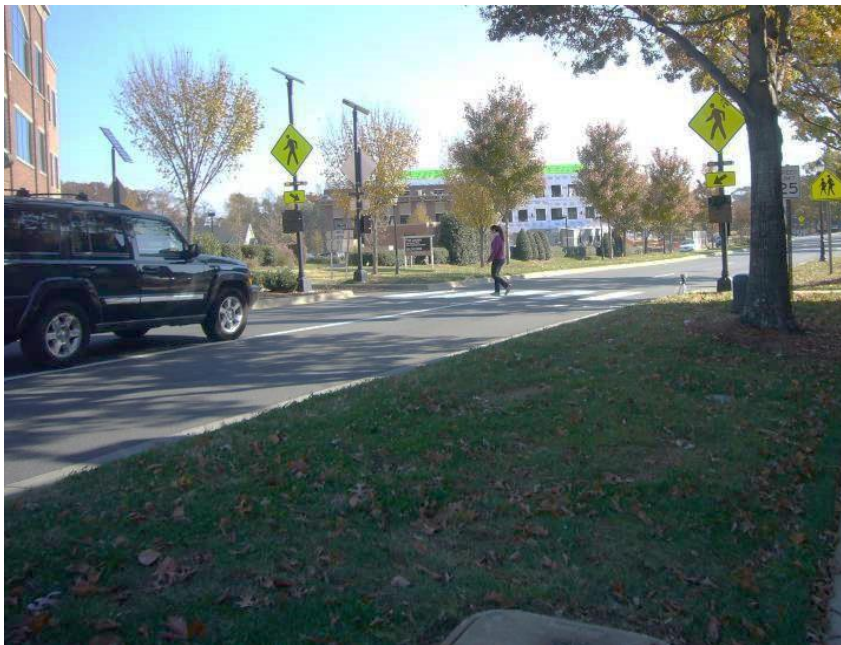
Figure 10-3: RRFB at Two-Lane Roundabout
