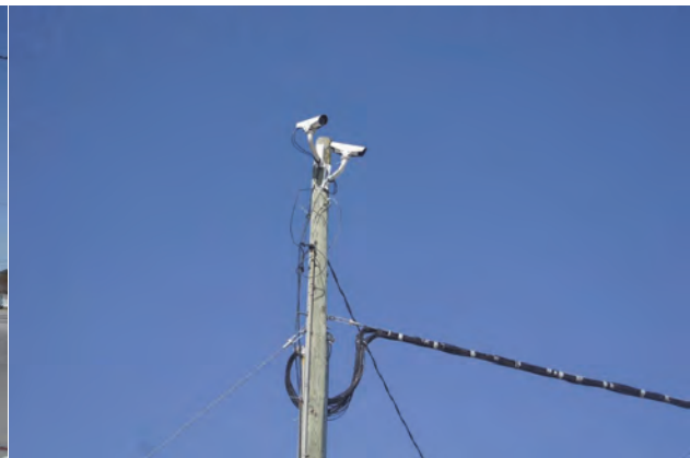
(b) Mounted Cameras on the Power Pole
