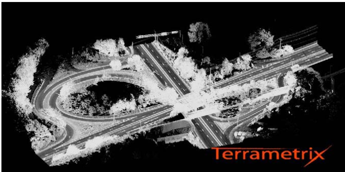
Figure 4.4. View resulting from dynamic multi-directional scanning
