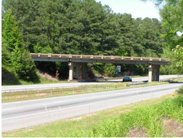
Figure 4.1. Bridge for SR 1010 over US 1 in Wake County.
