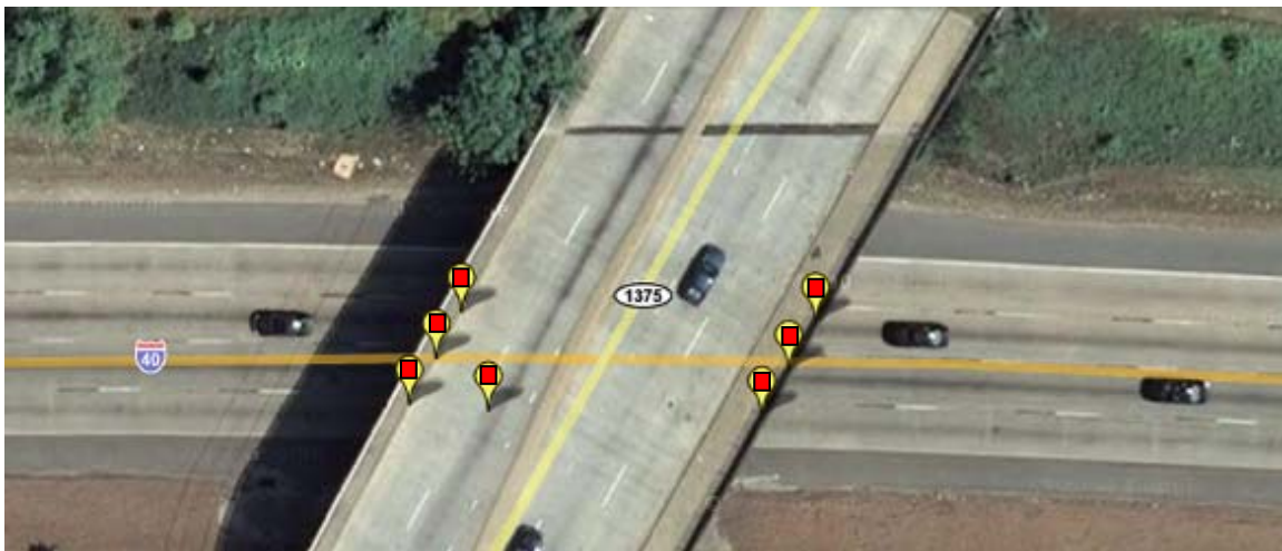
Figure 4.16. Terrametrix measurement locations for Lake Wheeler Road bridge.
