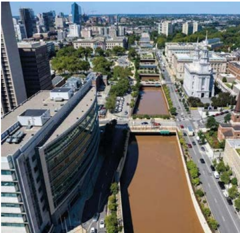
Hurricanes and other severe weather events can impact areas far inland from where they make landfall, such as seen here with flooding along I-676 in Philadelphia. (Credit: PennDOT)
