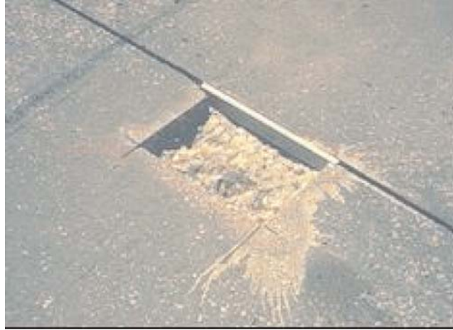
FIGURE B11 Prepared repair area; the insert, separating the repair area from the joint, extends beyond the saw cut into the existing longitudinal joint.
