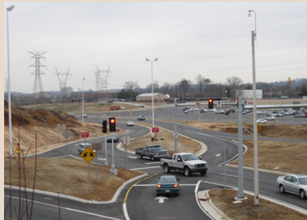
ITRE staff have been busy evaluating the operational and safety performance of Double-Crossover-Diamond (DCD) interchanges in collaboration with civil engineering at NCSU as part of a FHWA project.
