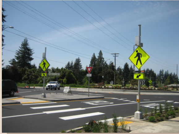
Rectangular Rapid Flashing Beacon (RRFB) is installed and evaluated on its ability to provide more yielding opportunities for pedestrians to cross as part of TOPR No. 34 project.
