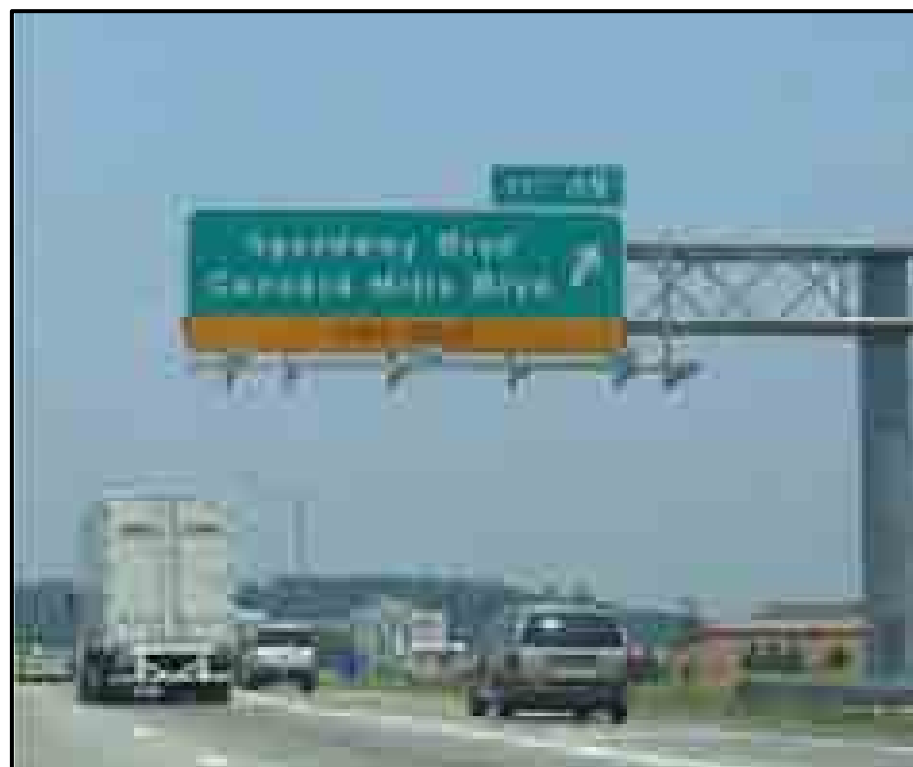
Exhibit 56: Overhead Traffic Signs
