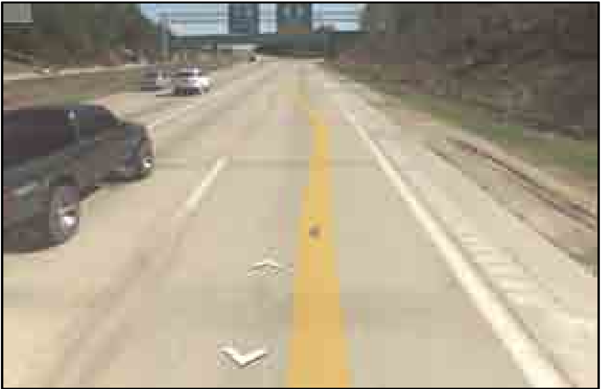
Exhibit 35: Example of transition zone, 4-lane facility drops two lanes. Vehicle must merge over 2 lanes to stay on loop (courtesy Google Earth).
