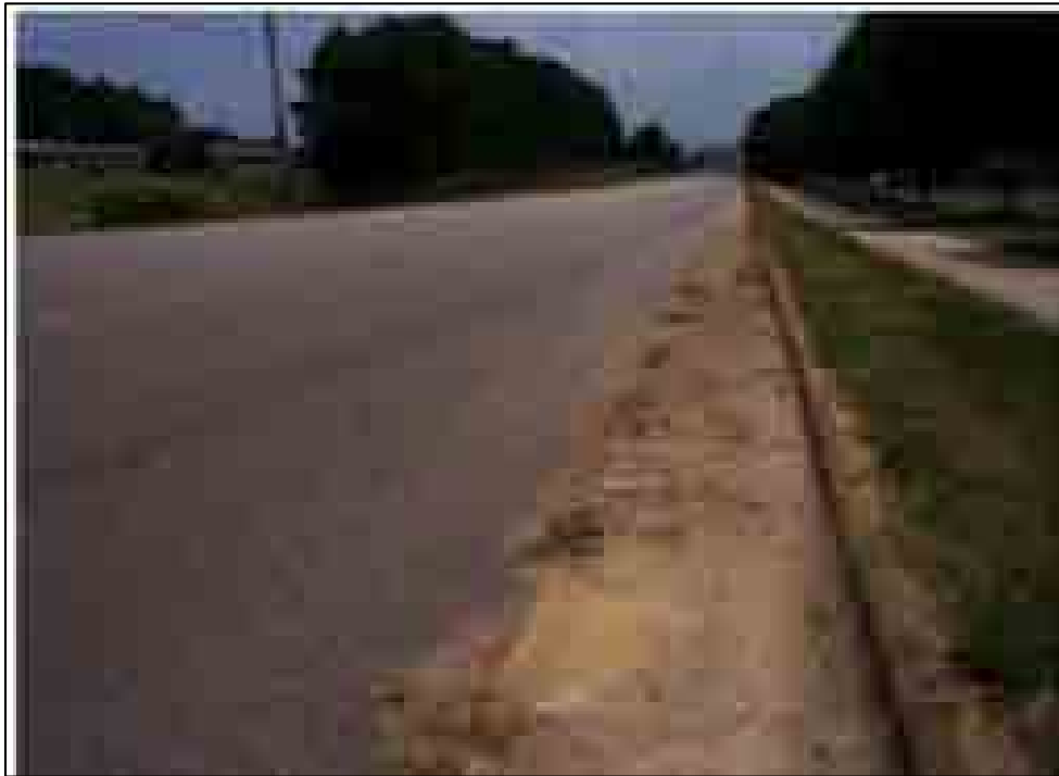
Exhibit 11: Curb/Gutter Blocked
