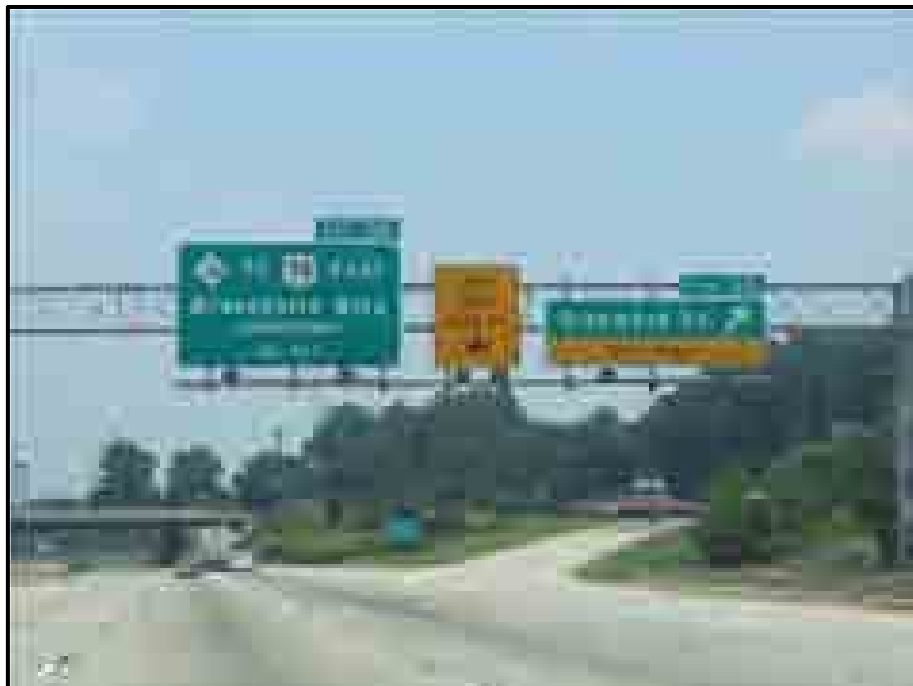
Exhibit 55: Overhead Traffic Signs
