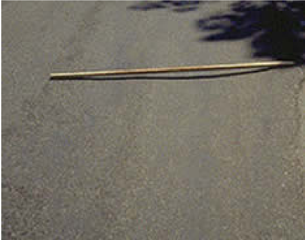
Exhibit 25: Rutting of Pavement
