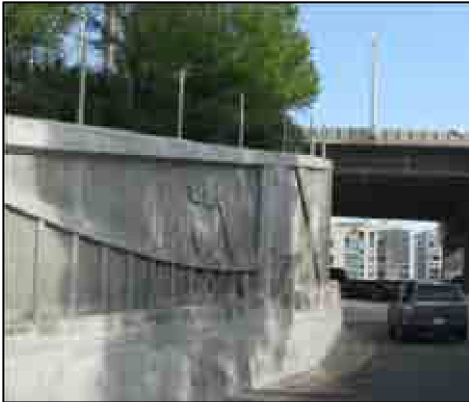
Exhibit 31: Retaining Wall– No Field Inspection Required
