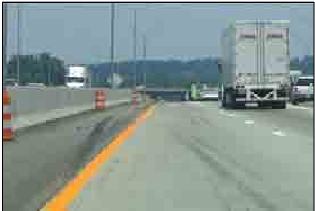
Exhibit 40: Pavement Marking – Skip Lines & Centerline
