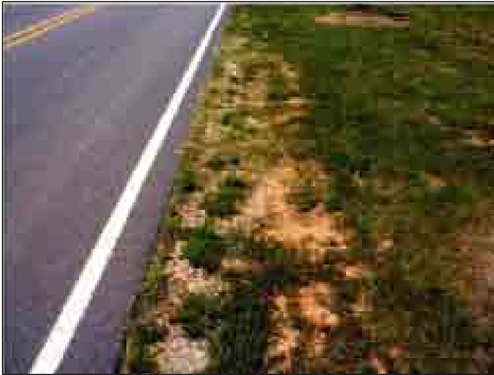
Exhibit 17: Turf Condition – Eroded/Bare
