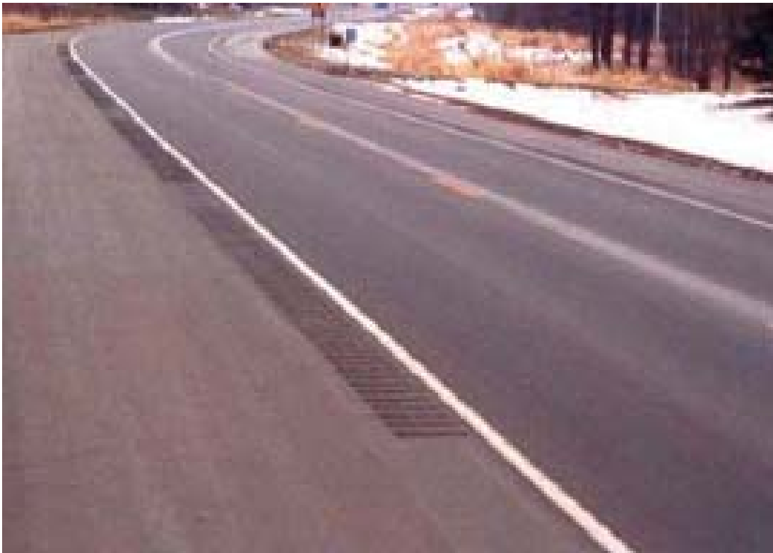
Exhibit 38: Gapped Rumble Strips along the travelway.
