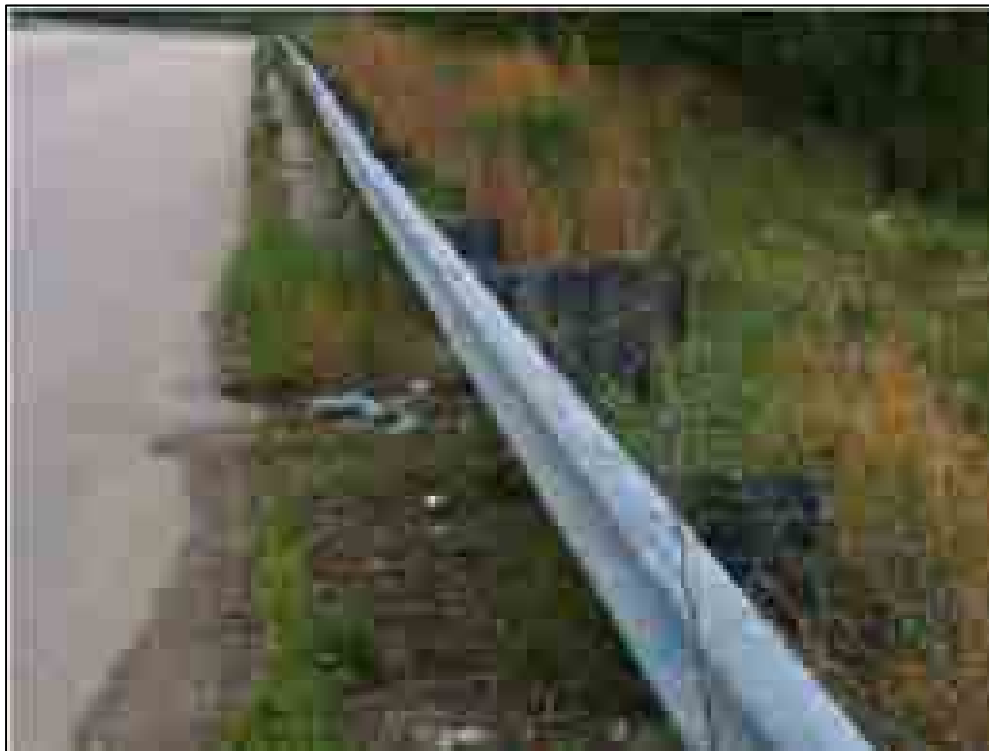
Exhibit 12: Curb/Gutter Blocked
