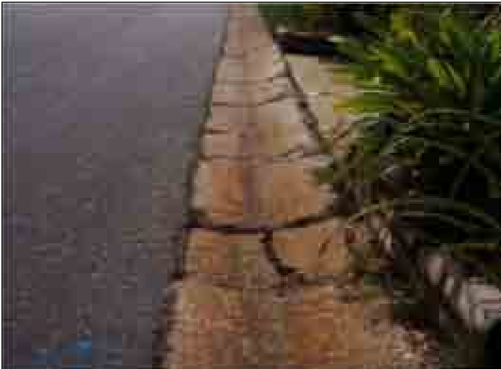
Exhibit 14: Curb/Gutter Damaged
